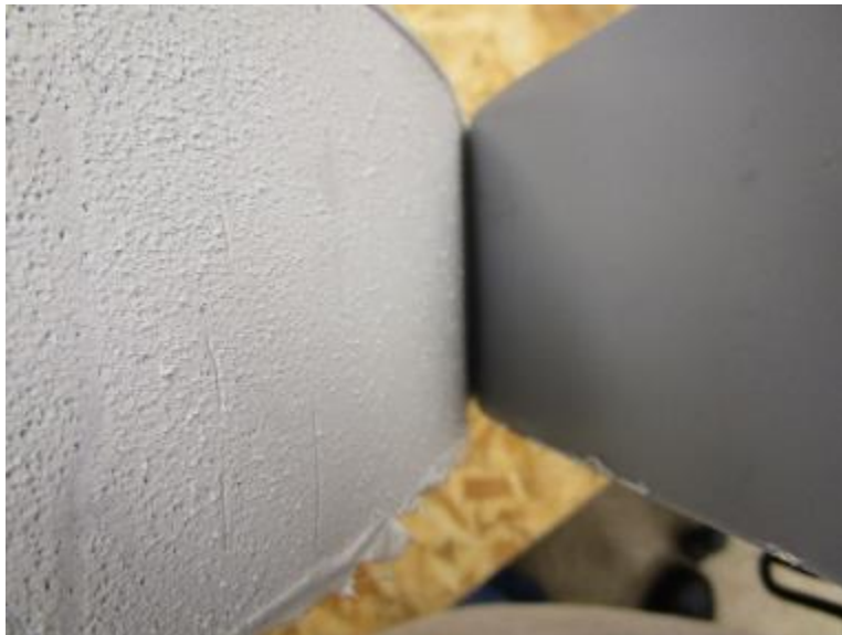
Photo No. 6 Typical Adhesion to Skin Failure Detail
